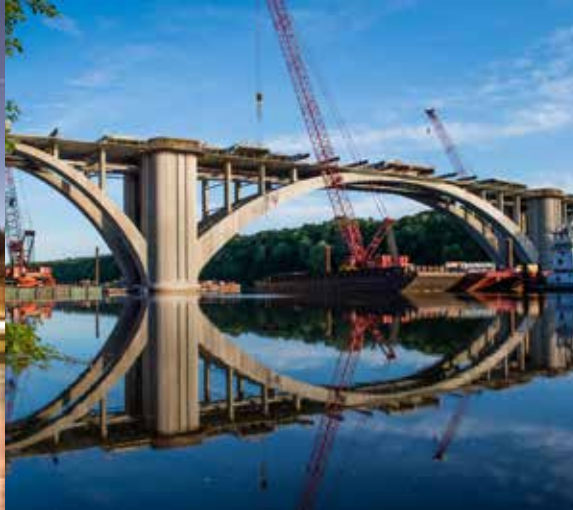
HIGHWAY & TRANSPORTATION RENOVATION
